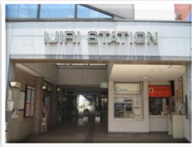
井尻 "Ijiri" Station
